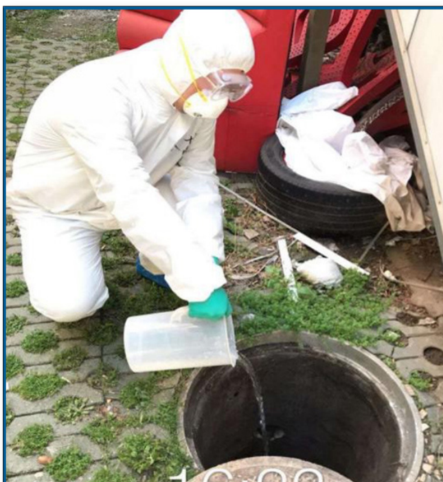
Disinfecting sewage systems.
